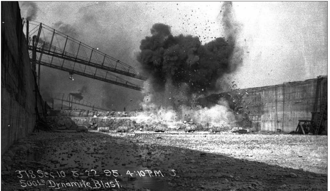
COURTESY OF METROPOLITAN WATER RECLAMATION DISTRICT OF GREATER CHICAGO
