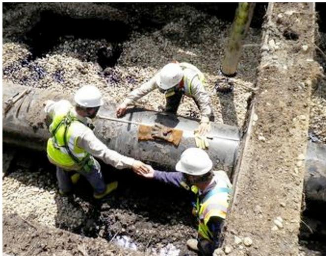
Technicians prepare pipe before cutting and removing the section from the Enbridge pipeline oil spill site near Marshall, Mich. Credit: EPA
